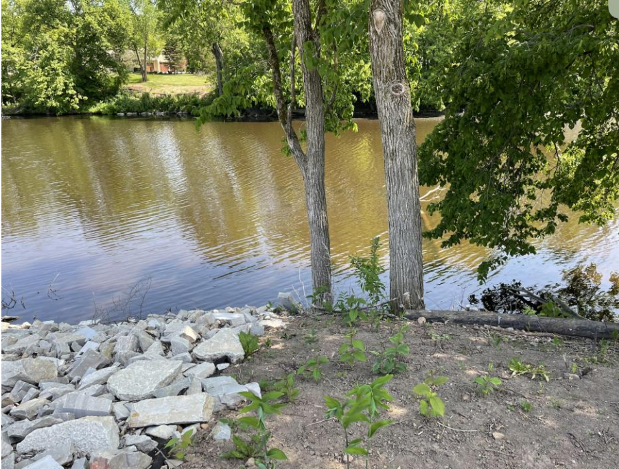
Riverbank, part natural and part riprap to prevent erosion.
